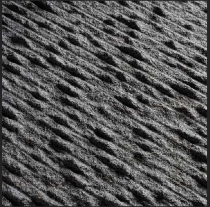
CUT BROKEN SAND BLAST
